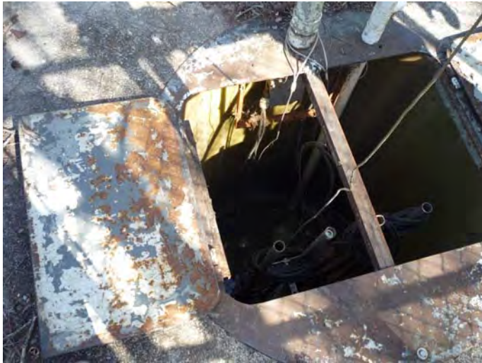
Valve Vault - Corrosion
