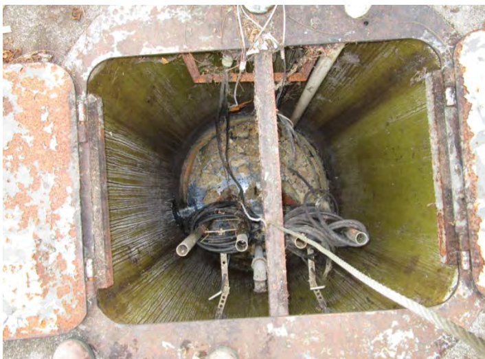
Fiberglass Wet Well
