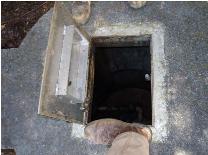
Undersized Valve Vault Hatch
