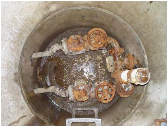
Valve Vault - Corrosion
