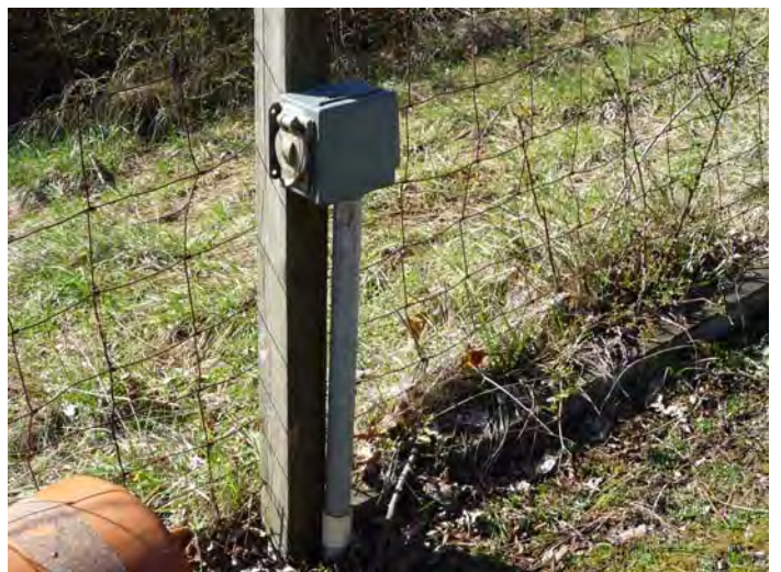
Emergency Generator Connection
