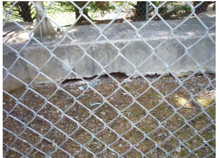
Undermined Concrete
