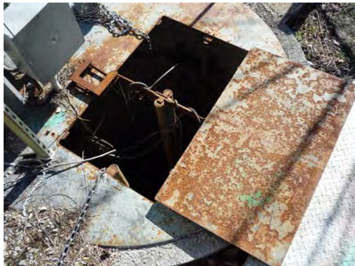
Wet Well – Hatch (Corrosion)
